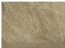
Vinyl Flooring Upstairs bathrooms
