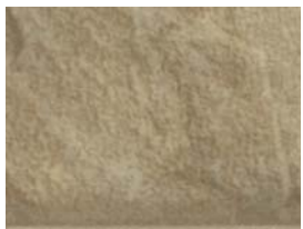
Vinyl Flooring Rear bath
