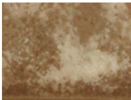
Vinyl Flooring Rear bath
